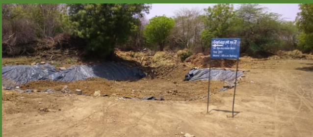
Garbage pit no.-7 when half full of bio-non-degradable garbage leveled and earth refilled.
